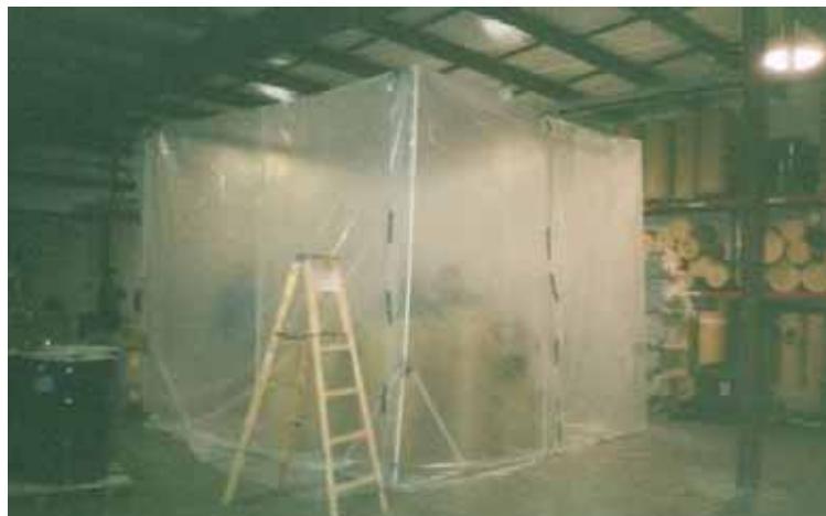
Photograph 2.1: AERC Ashland Facility - Containment Structure - First Visit
