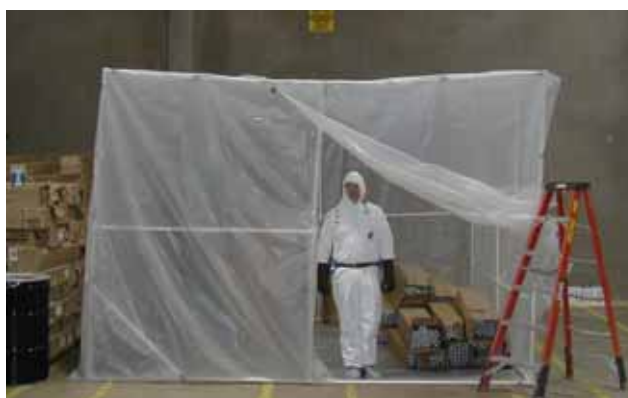
Photograph 2.2: EPSI Phoenix Facility - Containment Structure
